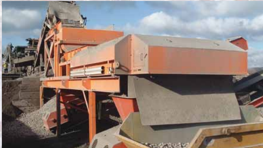
ECS Module at a steel producing plant
